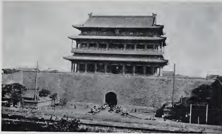
The Chien Men, main gate of the City of Peking, now an avenue of approach for all the world.
